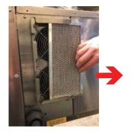
Remove the **two** air filters from the back side of the oven, one per side.
